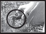
1. Insert ground rod next to the energizer. Then connect black clip to the ground rod (as shown above).
